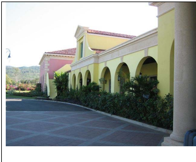
Picture 8.3 Sandals Whitehouse – Entry Elevation
