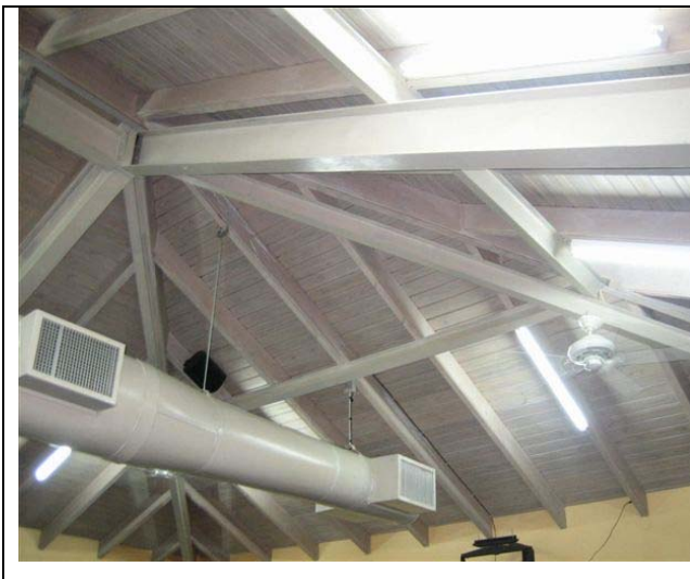
Picture 7-1 – Structural Steelwork support to timber roof
