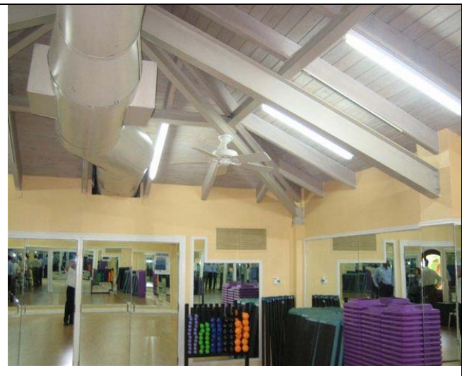
Picture 7-2 – Structural Steelwork support to timber roof
